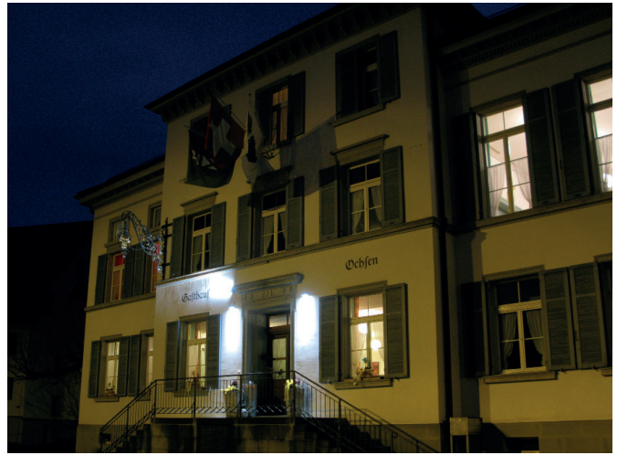
SpotLED 230V facade lighting
