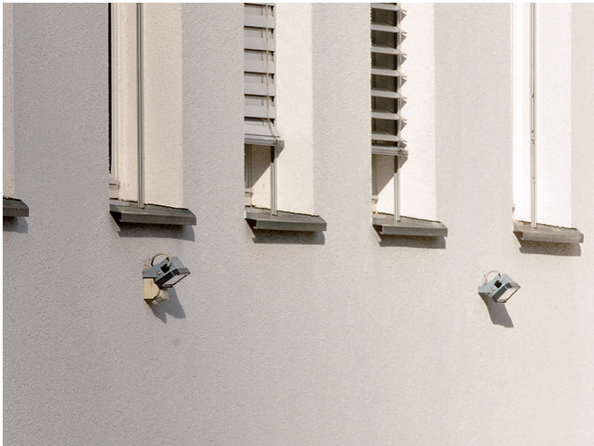
SpotLED 230 as outside illumination of municipal buildings
