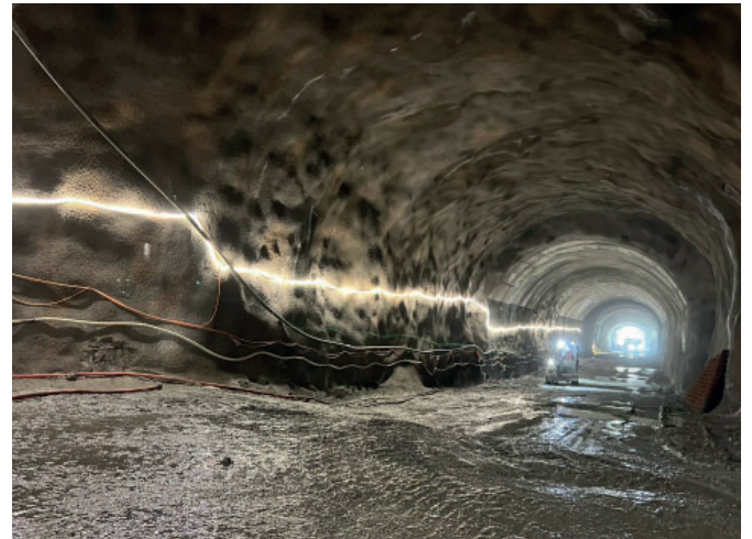
Implenia Switzerland, ARGE Gotthard
